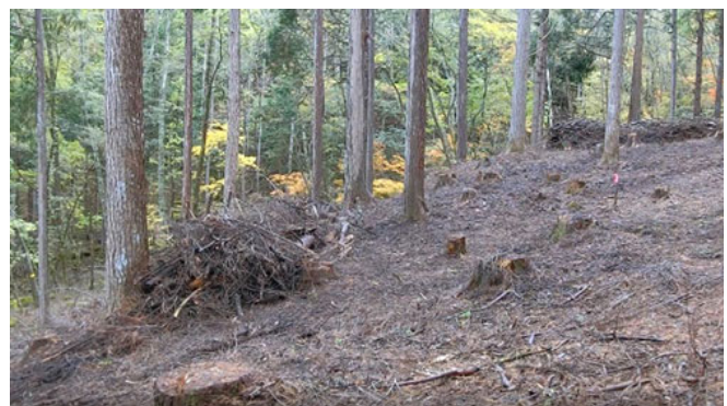
After site preparation: cleared ground where trees can be planted
