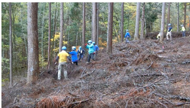
Site preparation: working by hand to gather up branches and foliage scattered on the ground
