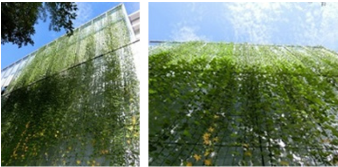
Green wall of vegetation at the Hachioji R&D Center
