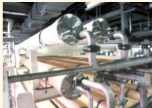
Kochi Casio's new facility to recover and reuse condensed water
